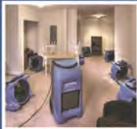
Structural Drying
